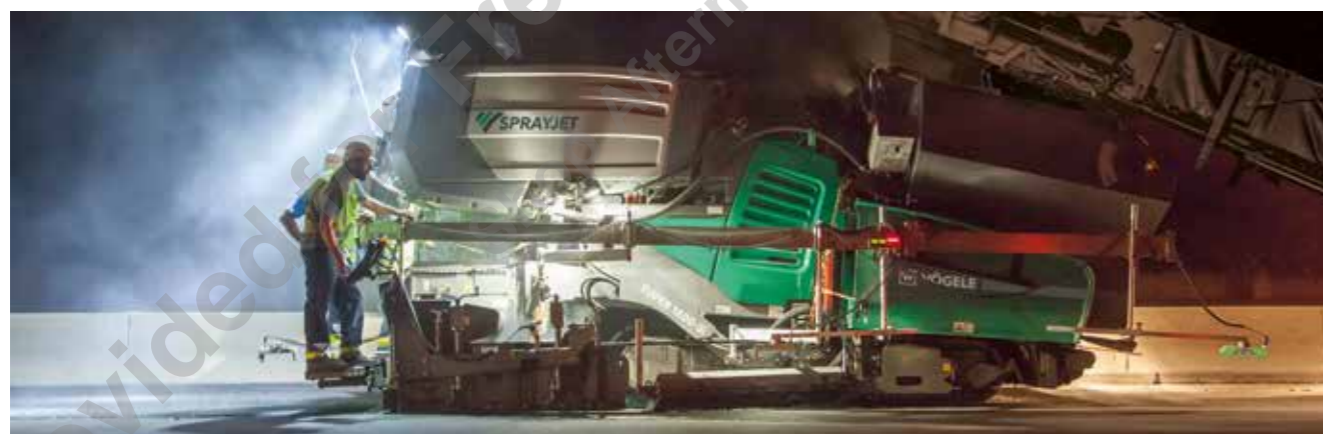
RESURFACING WORK ON A MOTORWAY
