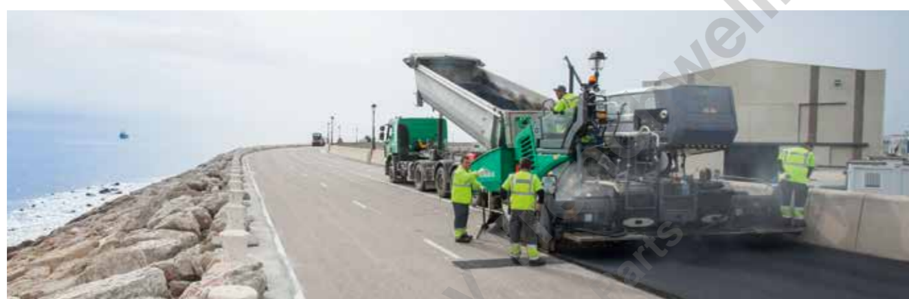
REHABILITATION OF A CAUSEWAY
